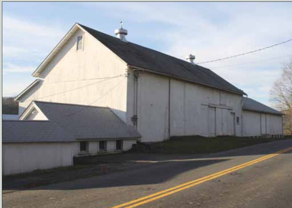
The Weantinoge Heritage Land Trust will be able to make repairs to the White Barn at the Smyrski farm in New Milford, thanks to a grant from The 1772 Foundation, administered by the Connecticut Trust.
