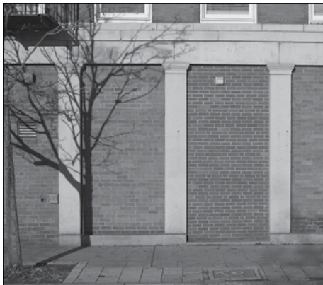
Part of the original granite-pier storefront survives on the Street Building.
