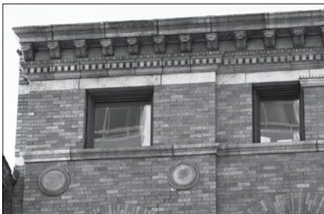
Ornamental masonry and cornice on the Monson Building.
