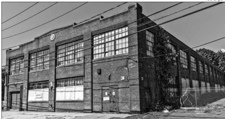
In 1921 the Norwalk Hour wrote that the Le Roy Shirt Company factory, "...presents an appearance that is both dignified and substantial and that comports with the solidity of the company and the reputation of the product."
