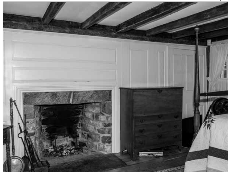
The evenly-spaced girders framing the Enos Kellogg house are a feature rare in Connecticut but more commonly found in the Hudson River Valley.
