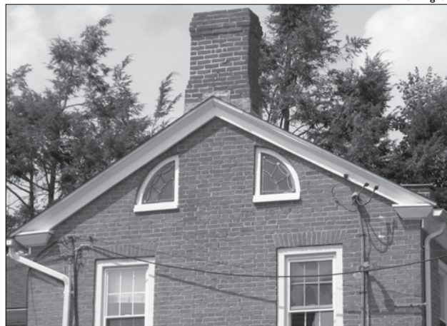
The Andrews-Olney house has fine Federal-style detailing.
