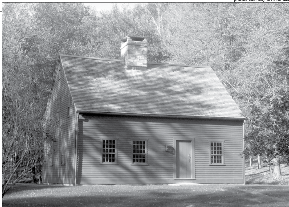
Restoration of the Turrill house included removing later additions and tracking down early woodwork and floorboards to replace lost originals.
