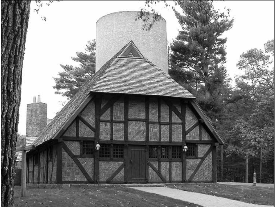
A grant will support needed repairs to the Water Tower, Forge, Chapel, and Smithy at Avon Old Farms School, designed by Theodate Pope Riddle to emulate a Cotswold village.
