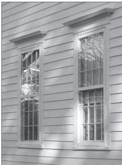
new storm windows installed
