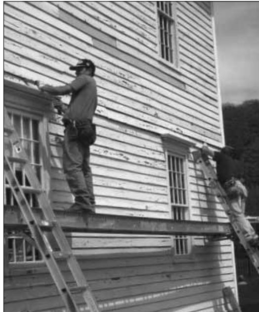
Repairs at the Whitney Boardinghouse
