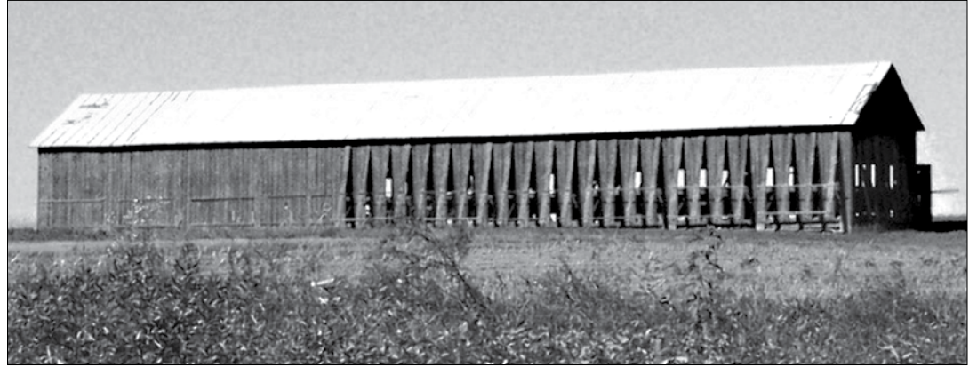
With its long, narrow shape and ventilation louvers, the tobacco shed is an instantly identifiable element of the Connecticut agricultural landscape.
