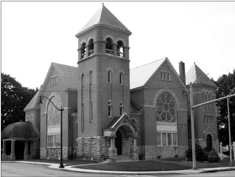
Norwalk: the former First United Methodist Church
