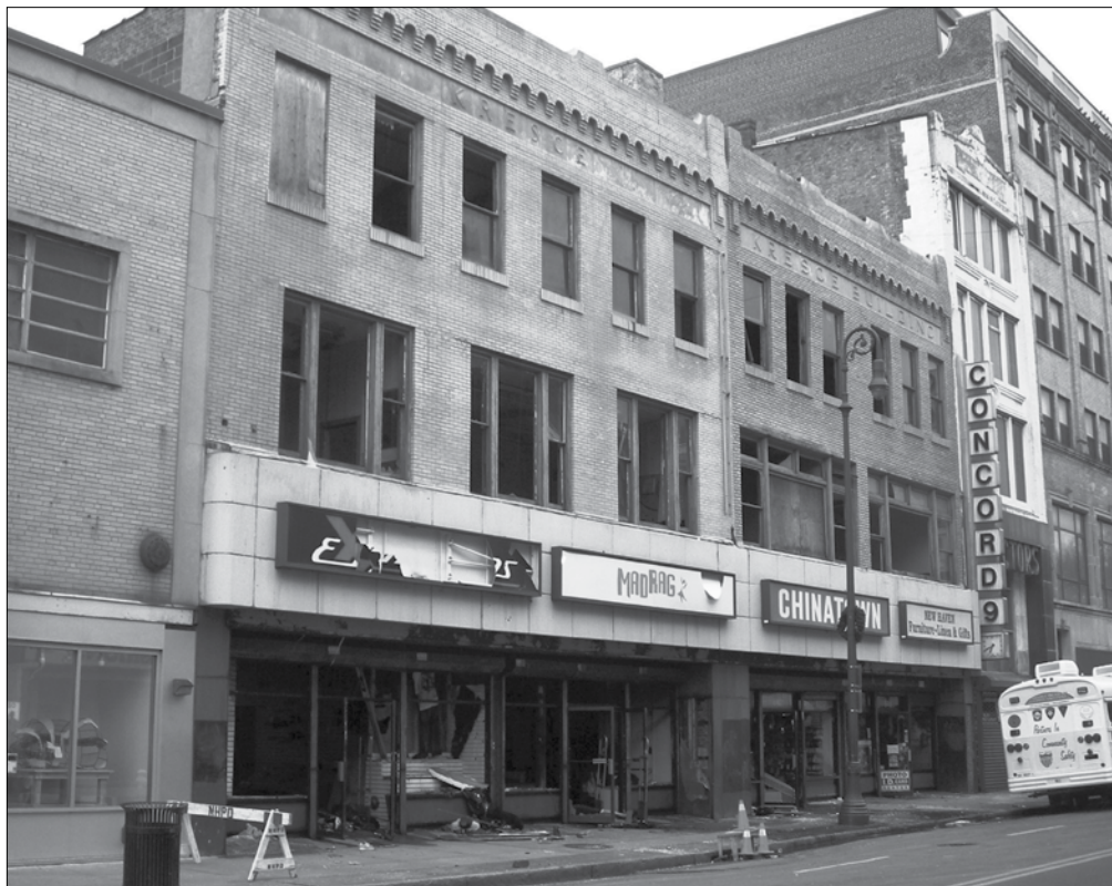
The Kresge Building in New Haven, damaged by fire in December.
