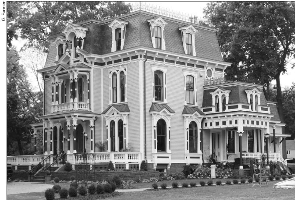
The Silas W. Robbins house, in Wethersfield, has been restored as a bed-and-breakfast
