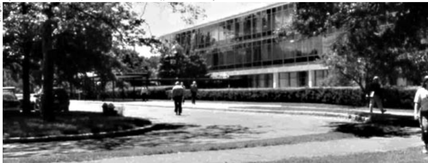
Cigna has announced plans to preserve and continue to occupy the Wilde Building in Bloomfield.
